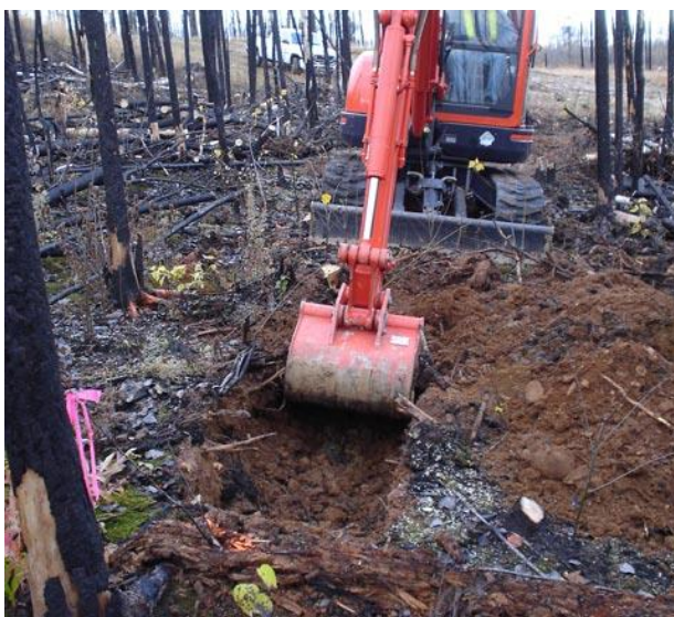
Figure 2-27: Excavation des tranchées © Terra Erosion Control
